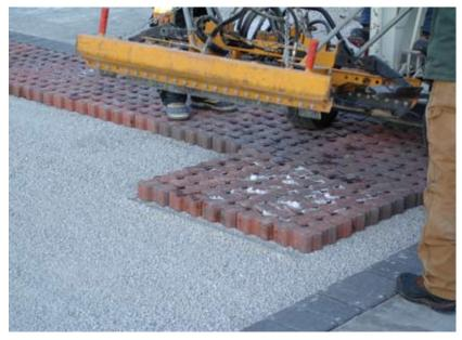
Figure 5. The permeable interlocking concrete pavers are supplied and installed in layers on the screeded bedding material, pea-sized aggregate (bedding sand is never used in PICP). Note the snow on the pavers doesn't interfere with installation and the border course against the concrete curb provides a finished edge.
