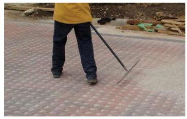
Figure 8. The paver openings are filled with the small stones (CA-16) and excess stones are removed from the paver surface prior to compaction.
