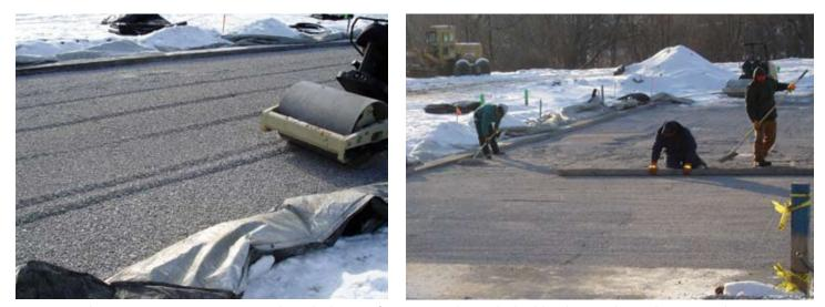
Figures 3 and 4. Compaction equipment completes the base surface prior to placing the bedding layer and screeding it smooth to receive the permeable pavers.
