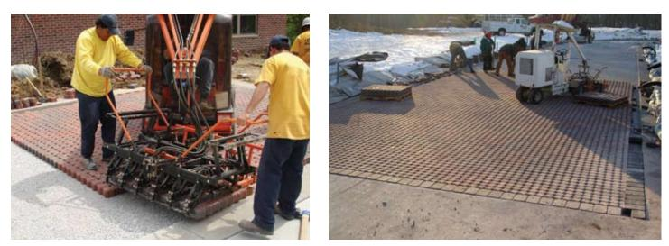
Figure 6 and 7. Mechanical installation equipment places ready-made layers of the concrete pavers. The equipment generally reduces paver installation time by 50% to 70% compared to manual installation.
